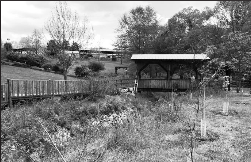
GMREC Repair and Planting in Progress at Creek Tributary
